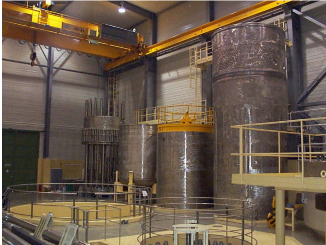
Figure 5: Real components as training objects at the Paks Maintenance Training Center
